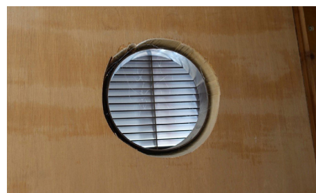
The fire door has had changes made to it after it was fitted, for example a ventilation grill has been added.
