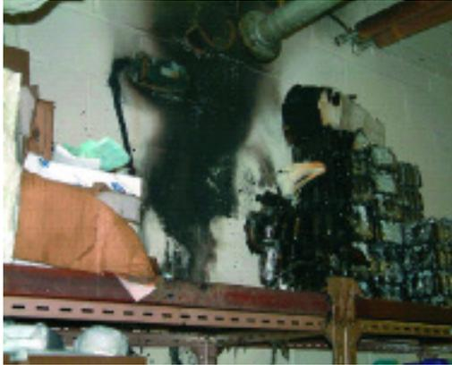
*Figure 4: Fire in a storeroom (hot works)
